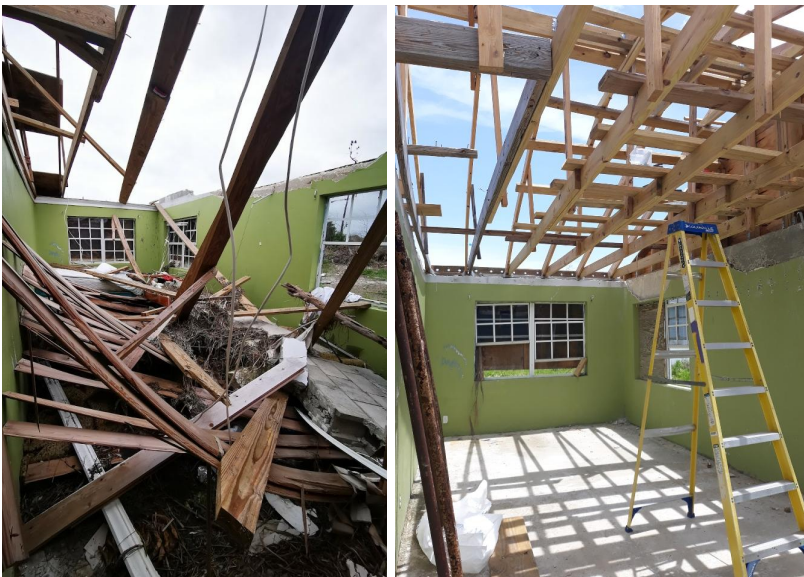
Wilson home after Hurricane Dorian (left) and current progress (right).
